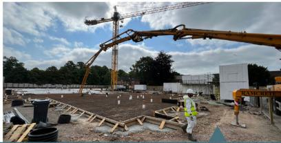
The primary objective was to enable the drainage to remain shallow due to the connections into the main runs outside the site. The slab thickness was kept to a minimum, with the shallow drainage combined within the slab where heave precautions were required.
