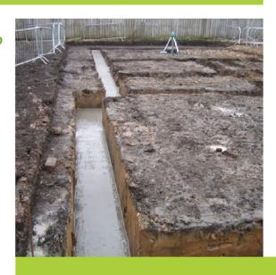
Dissolution features or voids in the subsoil pose a significant hazard to strip foundations.
