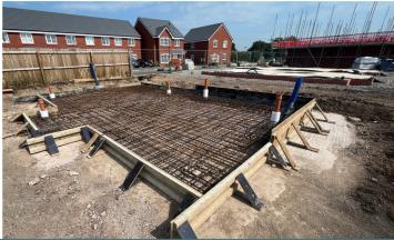
At Snelsmoor Grange, we delivered a full design-and-build piled raft foundation solution for 22 residential units and six garages. We overcame significant geotechnical challenges, including shallow clay soils, a high water table, and soft, saturated ground.
